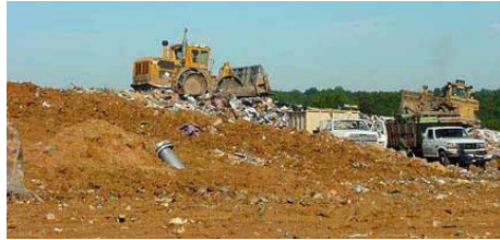
Landfills: Energy + Resources
